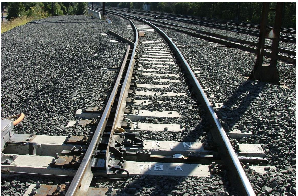
Figure 4 - Example of catchpoint with good landing zone
