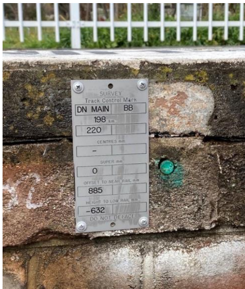
Figure 5 - Track Control Mark and Survey Plaque
