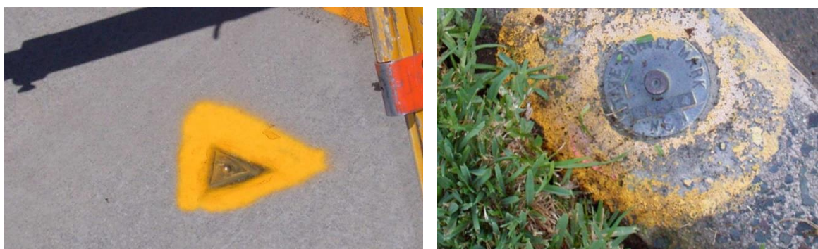
Figure 2 - Railway Survey Mark on Platform
