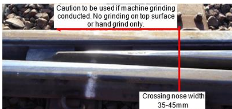
Figure 17 - Grinding of Crossing Nose
