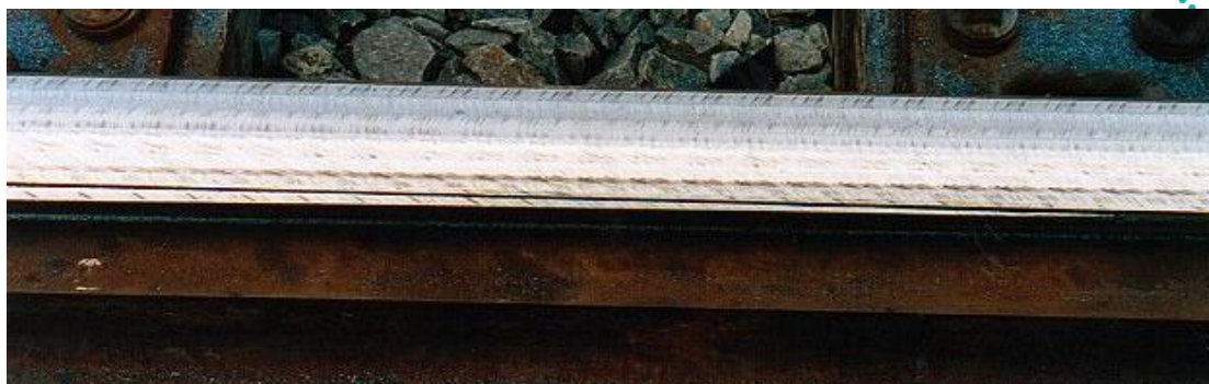
Figure 15 - Acceptable grinding finish at switch and stock rails
