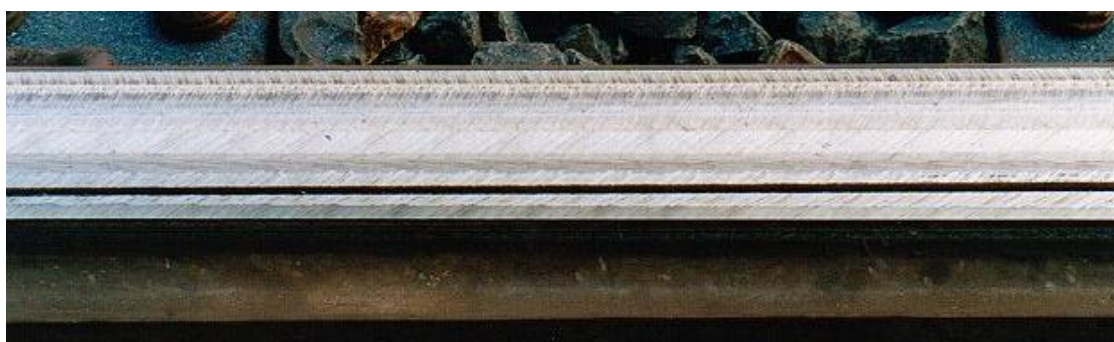
Figure 16 - Acceptable grinding finish at switch and stock rails
