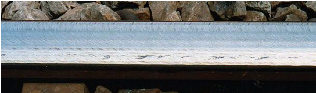
Figure 12 - Acceptable residual gauge corner defects after grinding
