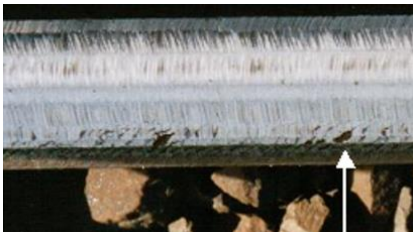
Figure 8 - Example of Gauge Corner Checking Defects Left in the Rails After Grinding (Arrow Points to the Gauge Corner)
