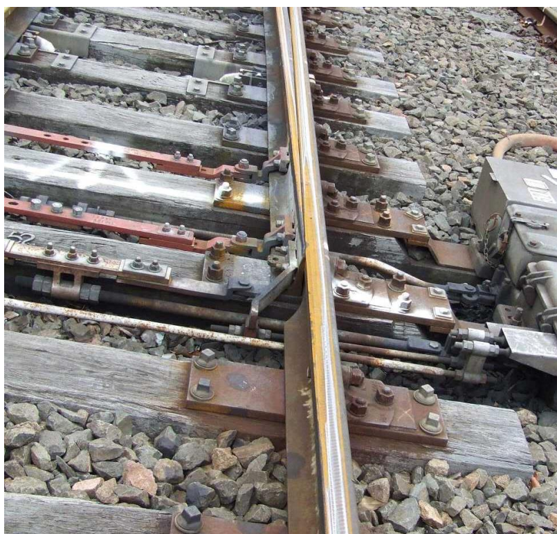
Figure 14 - Unacceptable excessive gauge corner grinding on the stock rail near the switch tip
